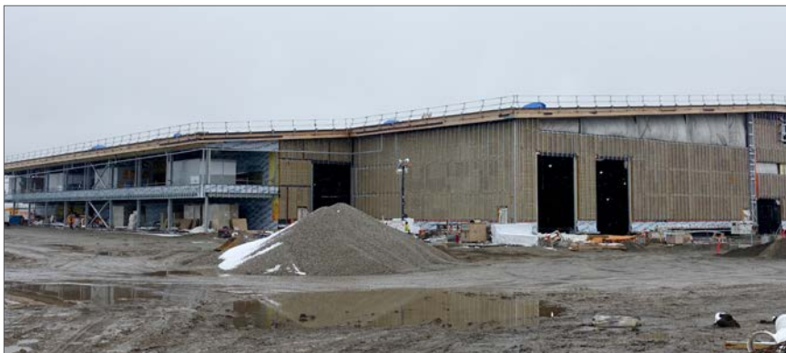
Gerry Wright Operations and Maintenance Facility - September, 2018
