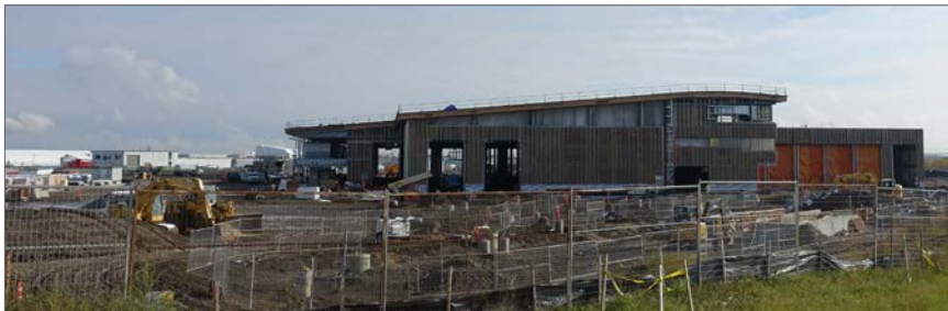
Gerry Wright Operations and Maintenance Facility - September, 2018
