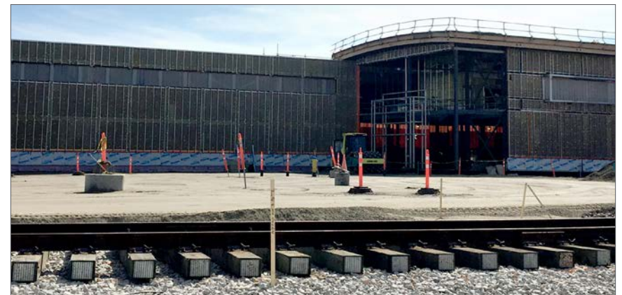
Gerry Wright Operations and Maintenance Facility - September, 2018
