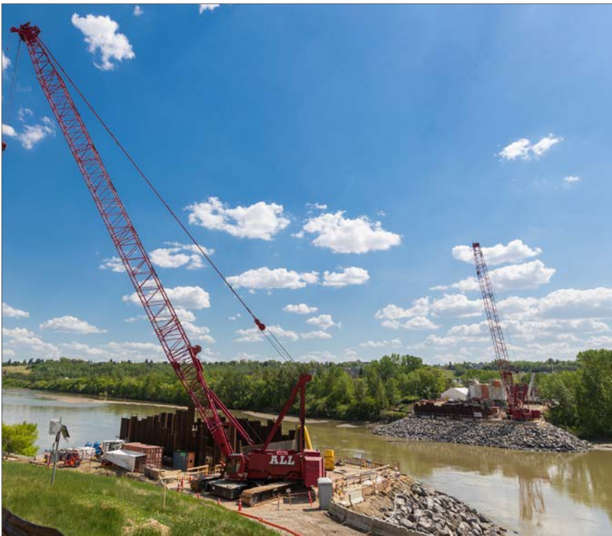
Coffer Dams - July, 2018
