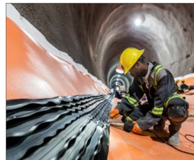
Tunnel Interior - July, 2018
